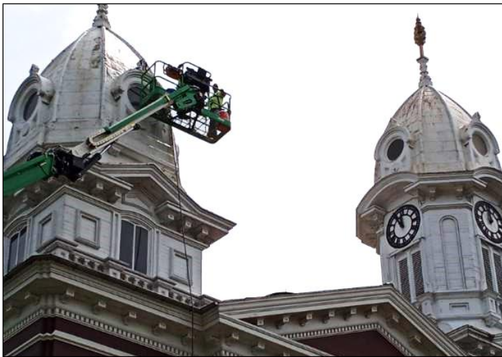
Tower Restoration - Before
