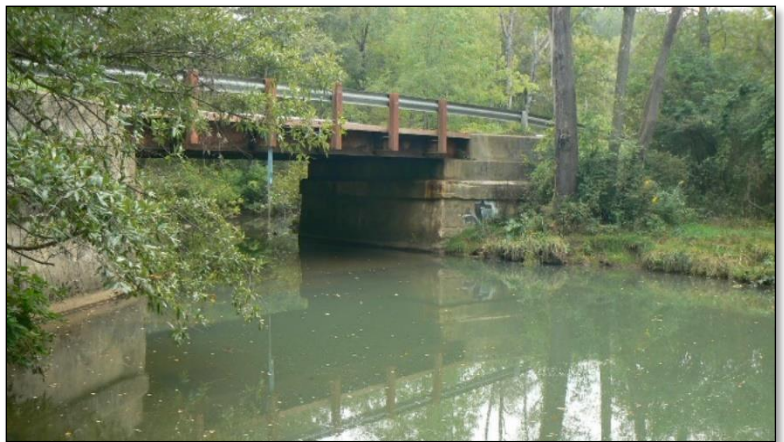
Aires Hill Bridge, Cranberry Township
