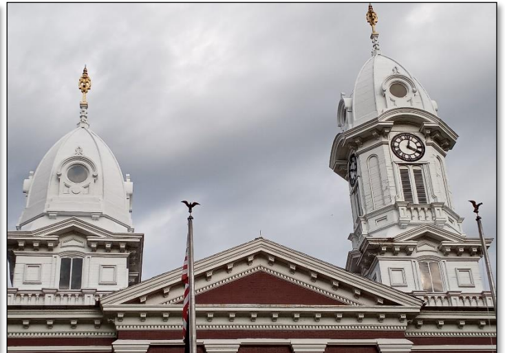
Tower Restoration - After
