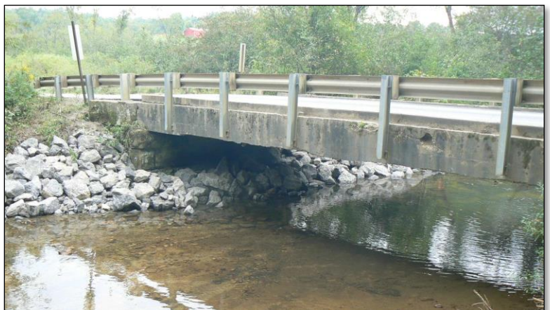
Old Beech Road Bridge, Irwin Township
